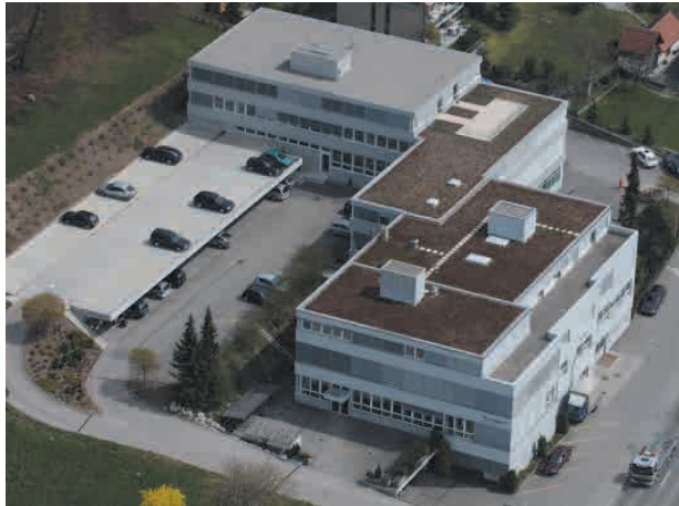
Headquarters in Orpund, Switzerland, Facility 1 瑞士总部
